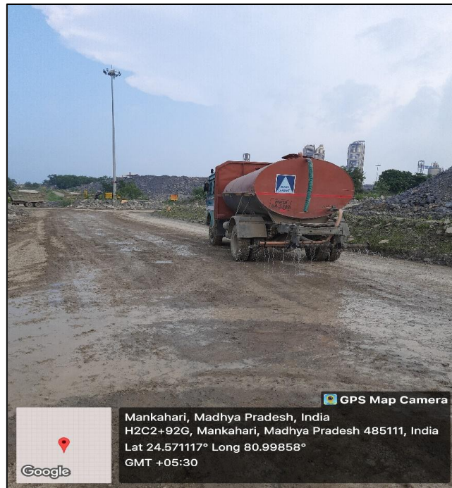
Water spraying done on the entire haul roads round the clock by water tanker
