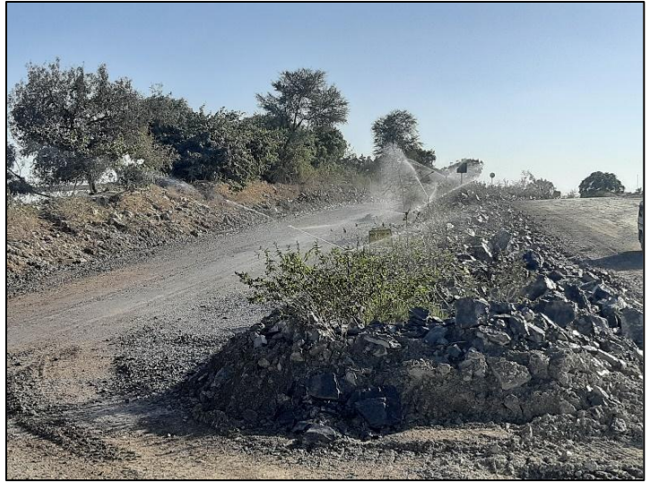
Permanent sprinkler arrangement along the haul road area
